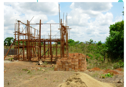
Guest House under construction. See story on page two.
