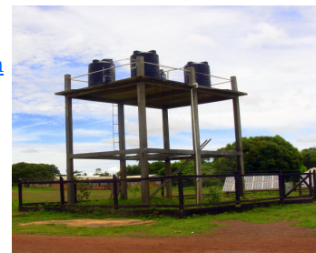
The current trestle
